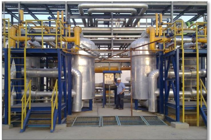
Nitrogen dryer 34 000 Nm 3 /h – 10 Barg
