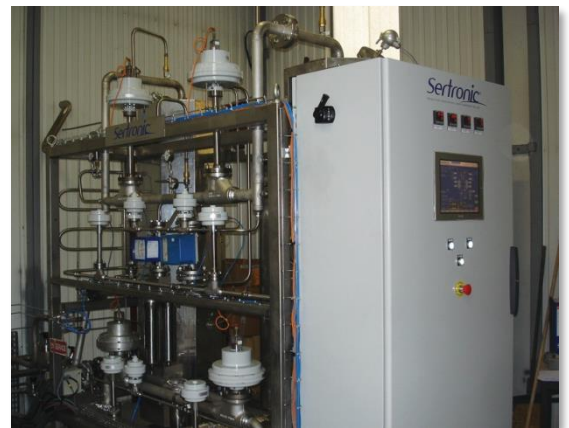
Nitrogen purifier N 500 – 15 500 Nm 3 /h – 15 Barg
